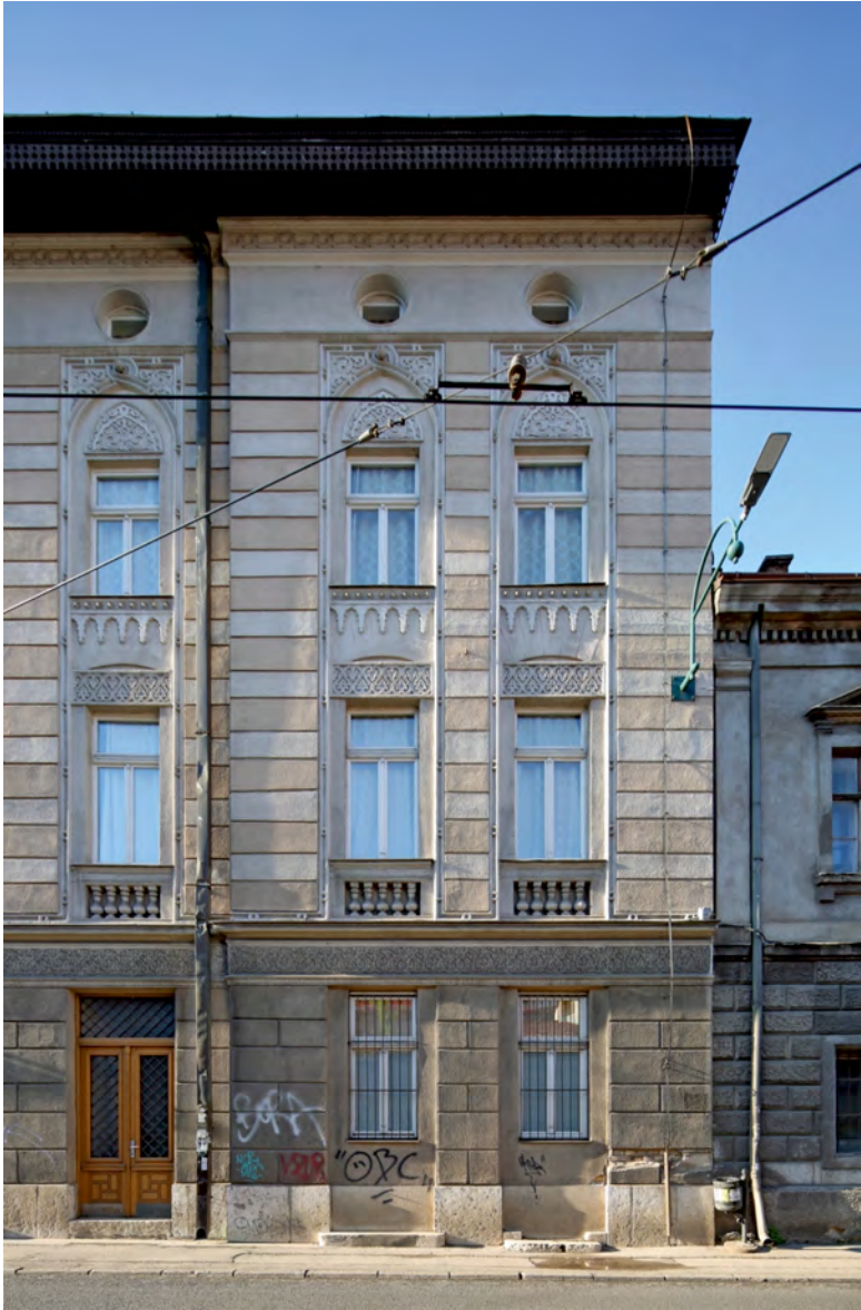
Fig. 1: Sarajevo, mixed-use building known as Đulagin dvor, 1896–97, Arch. Hans Niemeczek, photograph by Anida Krečo, 2023.
