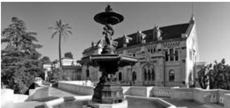
The main building of the University of Nice, Chateau Valrose. Photo: archive
