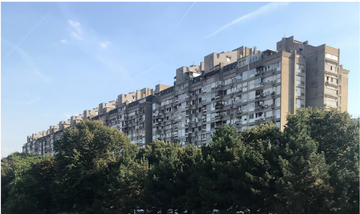
Figure 2. Photo of building no. 6, Block 23 in the present moment.
