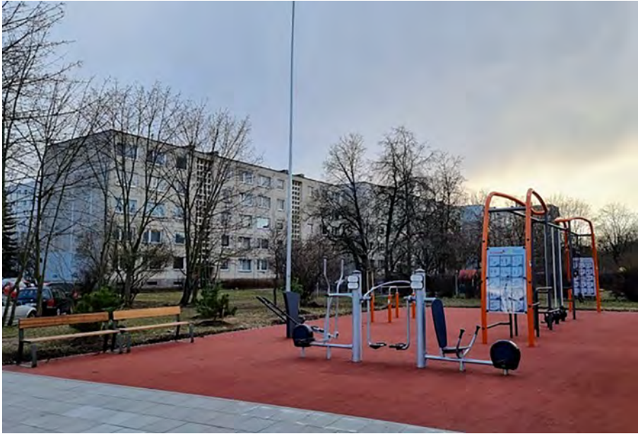
Figure 5: New sport facilities in Zirmunai triangle area, constructed with EU financial support.
