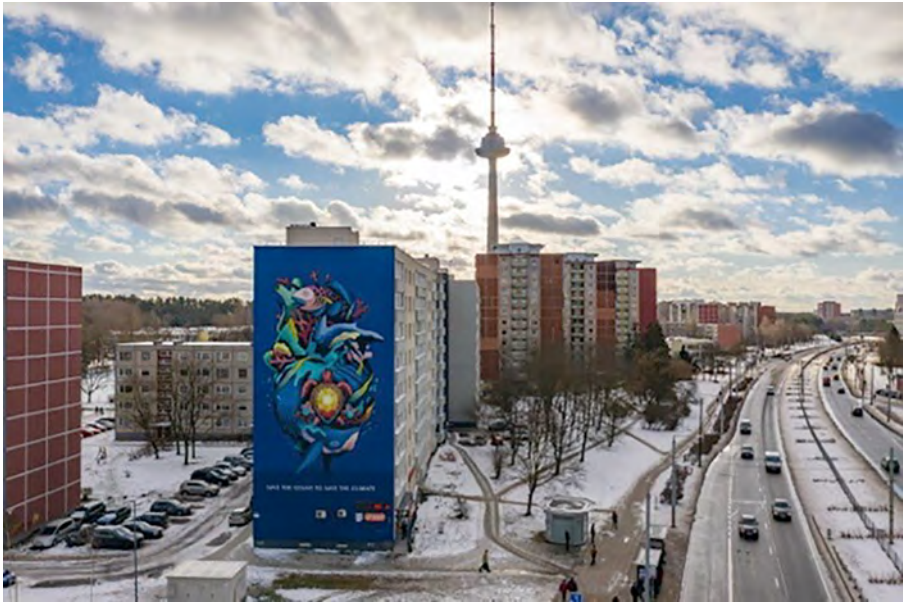
Figure 3: Street art creates new identity for renovated buildings.
