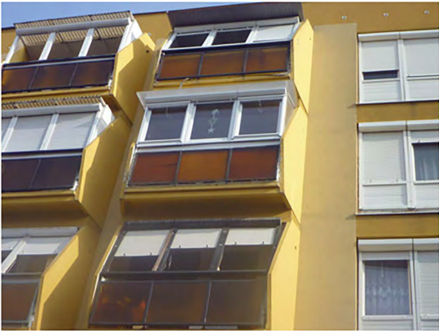
Figure 1: Informal balcony enclosures.
