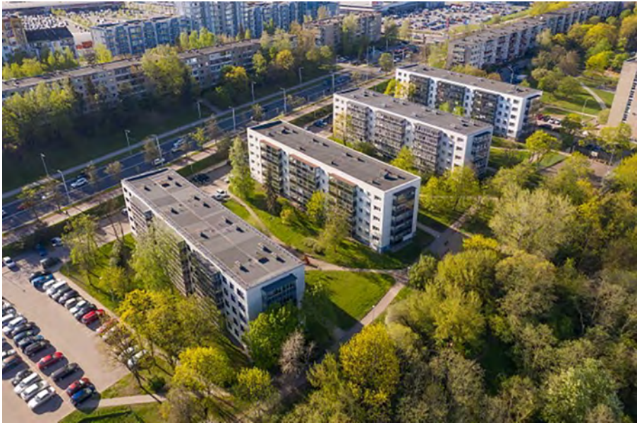
Figure 1: Newly renovated prefabricated buildings constructed between 1960 and 1970.
