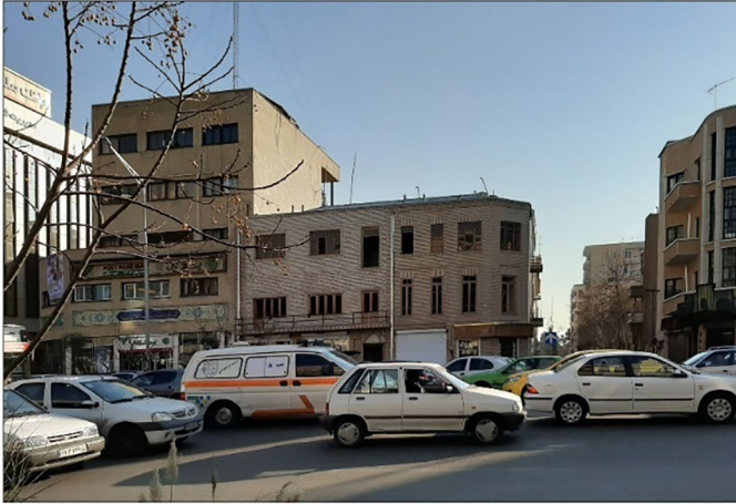
Figure 42: Examples of beautified facades in Enghelab Street
