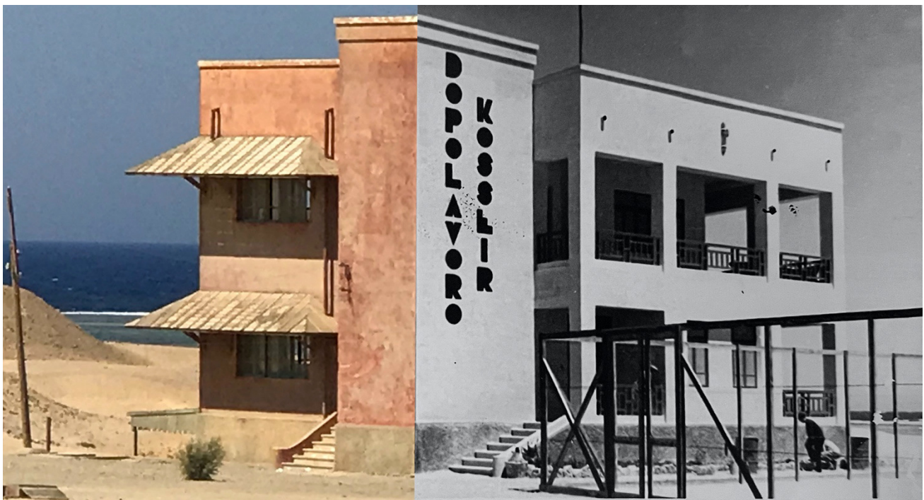
Figure 9. The cafeteria inside the coastal plant, where most scenes of the 2022 movie El-Gareema were filmed (left); the building was originally built as a restaurant, where Italians and Egyptians used to gather during lunchtime (right). Sources: Project fieldwork (2022; left) and Pellegrini (2011, p. 187; right).
