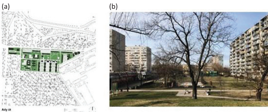
Figure 4. Ady HE: (a) Layout and (b) slabs built by the Danish Larsen-Nielsen (left) and Soviet-type (right) panel technology.
