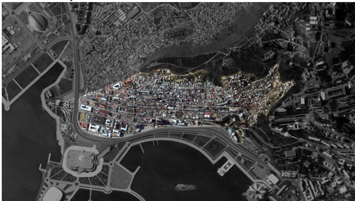
Picture 1: Bayil Is a Settlement Of Sabayil District With Low-Rise Buildings Located On a Steep Landscape.
