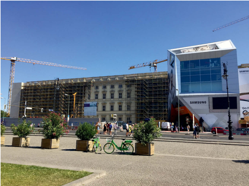
1.1 Humboldt Forum under construction, July 2018. Photograph by Sharon Macdonald.
