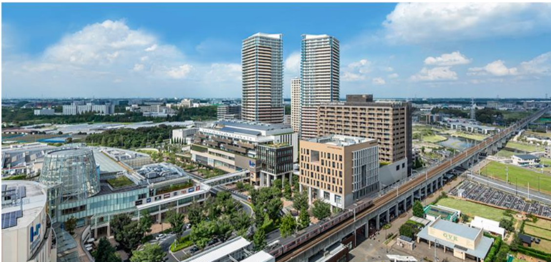
Figure 3 Skyline of Kashiwa-no-ha Smart City in Chiba Prefecture, Japan (Source: Hitachi 2017).
