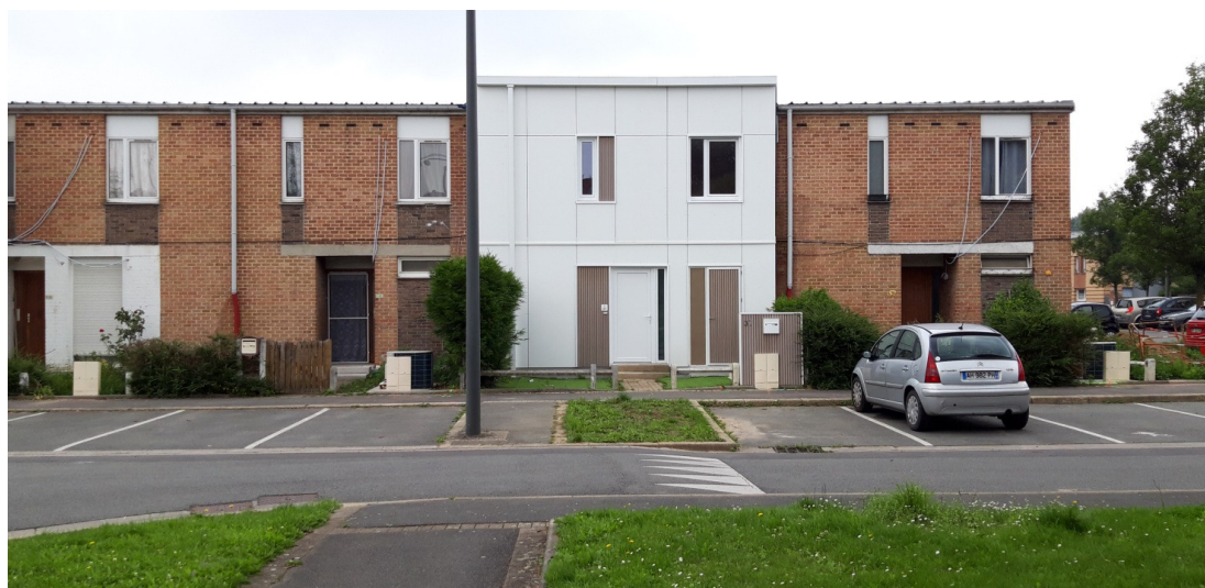
Figure 1. A prefabricated facade for a renovated house in Wattlelos.
