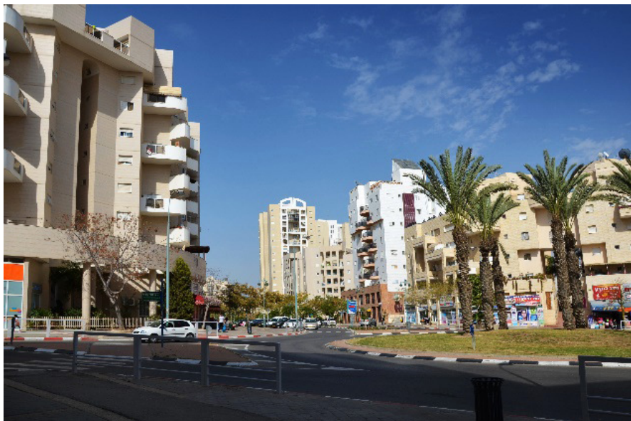
Figure 7. Mixed-use main axis in Neve Zeev Neighborhood, Beersheba, by AMAB Architects (1990s). Each building was planned by a different architect.
