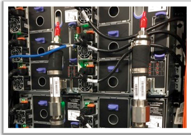
Figure 18: Fluid elements running through the system. Vertical tubes for water, black cables for electricity and blue for information. Source: Own photo
