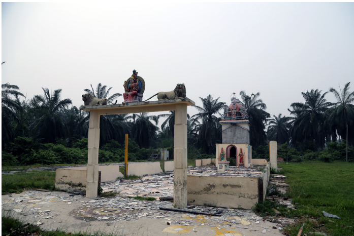
Figure 1. The demolished estate temple. This was my first sight of the demolished temple during the first day of revisiting. (Photo taken during fieldwork).
