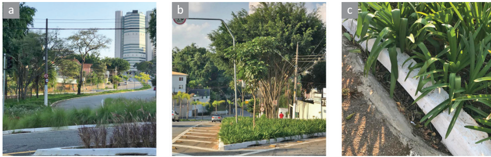
Figure 6. Programa Gentileza Urbana: Interventions in São Paulo; (a) overview of street with rain gardens; (b) a rain garden at the intersection of two streets; (c) kerb detail for water flow.
