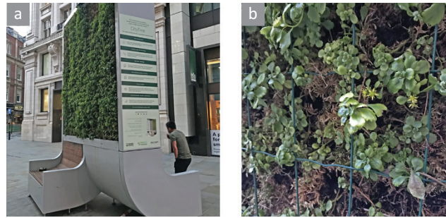
Figure 7. CityTree moss vertical infrastructure in London: (a) general view; (b) detail of moss and plants arrangement.
