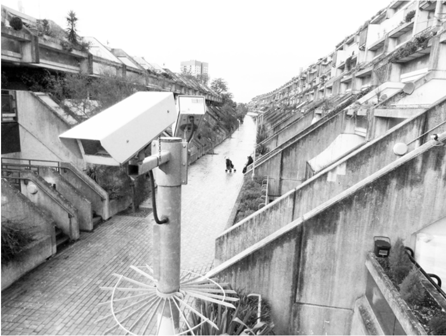
Figures 5 and 6: Spatial intersection of two discourses respectively two 'regimes of practices': Disciplining and surveillance on the one hand, appropriation and everyday use on the other hand. Alexandra Road Estate, designed by Neave Brown of Camden Council's Architects Department in 1968, constructed between 1972 and 1978. London 2011
