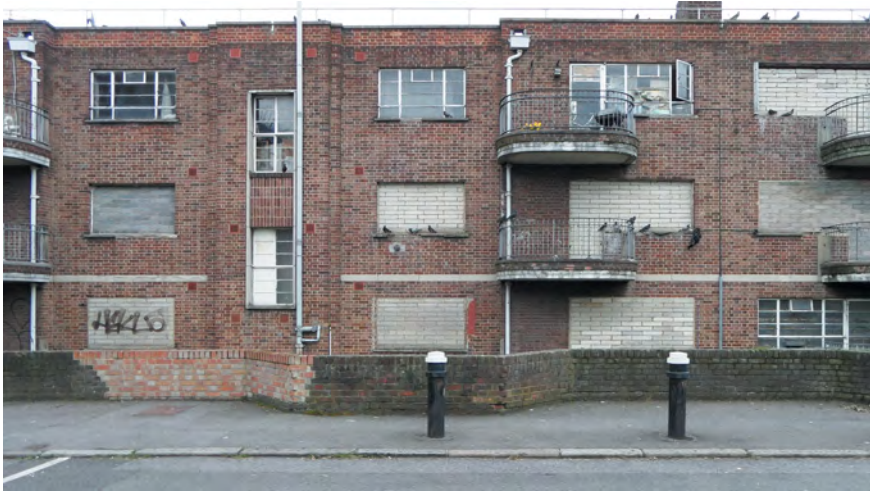
Figure 17: Obsolescence and creative destruction at work in Haggerston, London Borough of Hackney. The Kingsland Estate, built in 1949, is prepared for demolition after the majority of the residents voted in favour of urban renewal in 2007. East London 2013
