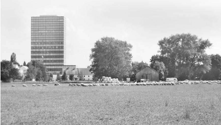
Figure 26: Unexpected coexistences in the 'Zwischenstadt'. High-rise 'capsule' Süddeutsche Verlag building, designed by GKK Architekten in 2008, and grazing sheep, East Munich 2017
