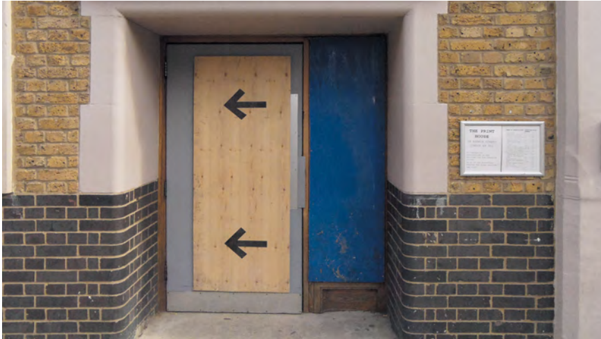
Figure 23: Boarded-up entrance to Print House during violent protests against inequality, racism and urban marginalisation in London and other British cities. The building is managed by the community-based, not-for-profit Bootstrap Charity. Dalston, London Borough of Hackney 2011
