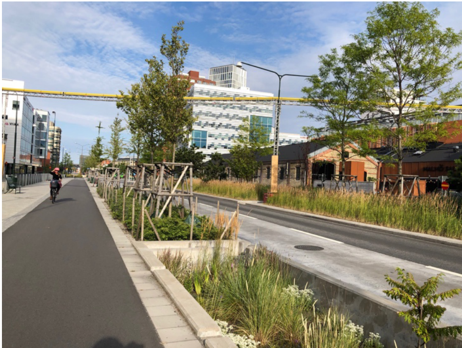
Figure 4. Central Malmö, Sweden: Biophilic streets with water sensitive urban design plus stratified street tree planting. Source: Authors.
