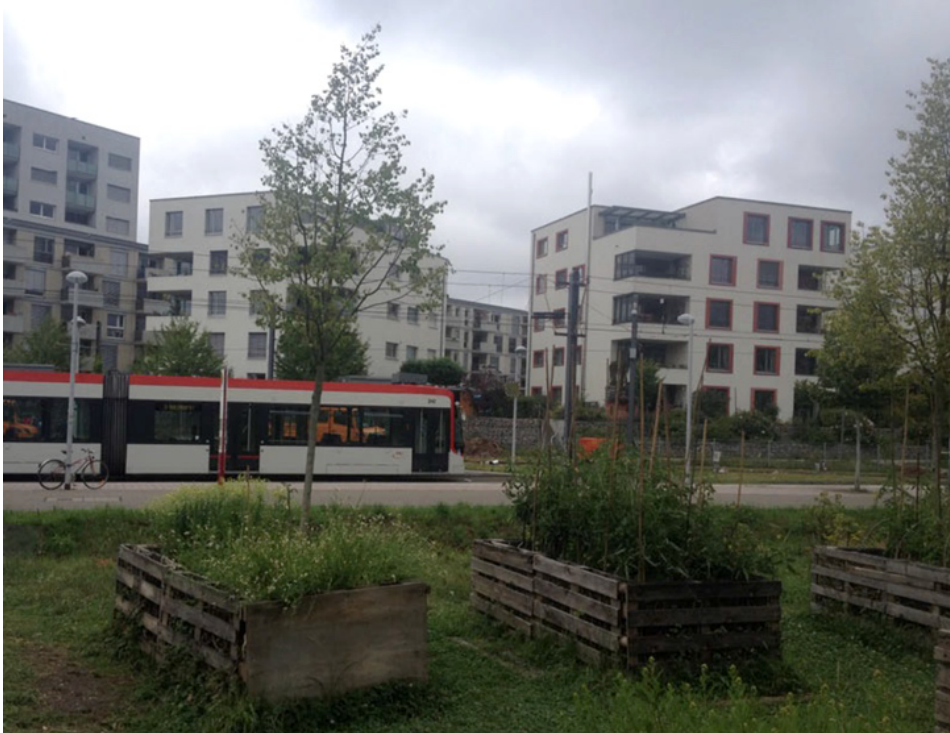
Figure 5. Vauban, Freiburg, Germany, a medium density transit urban fabric serviced by tramline with lawn base to mitigate noise and allow water infiltration surrounded by multiple house-based biophilic features. Source: Authors.
