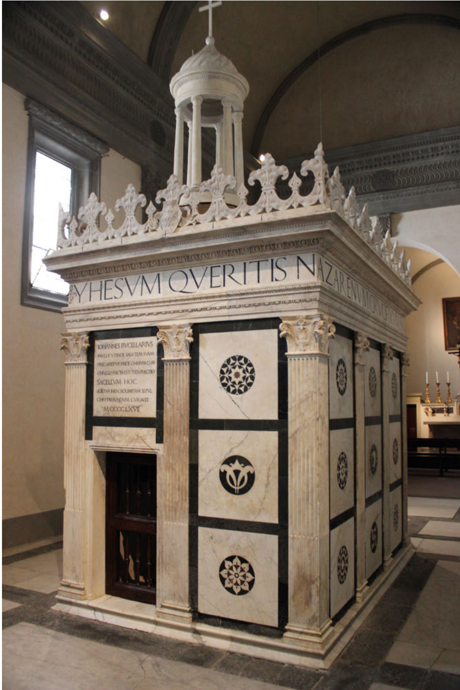
Abb. 28: Florenz, San Pancrazio, Capella Rucellai, Fassade.
