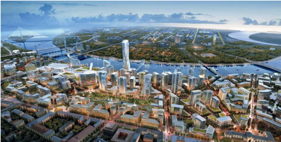
Fig. 2: Belgrade Waterfront project /Source: Belgrade Waterfront; https://www.belgradewaterfront.com/en/
