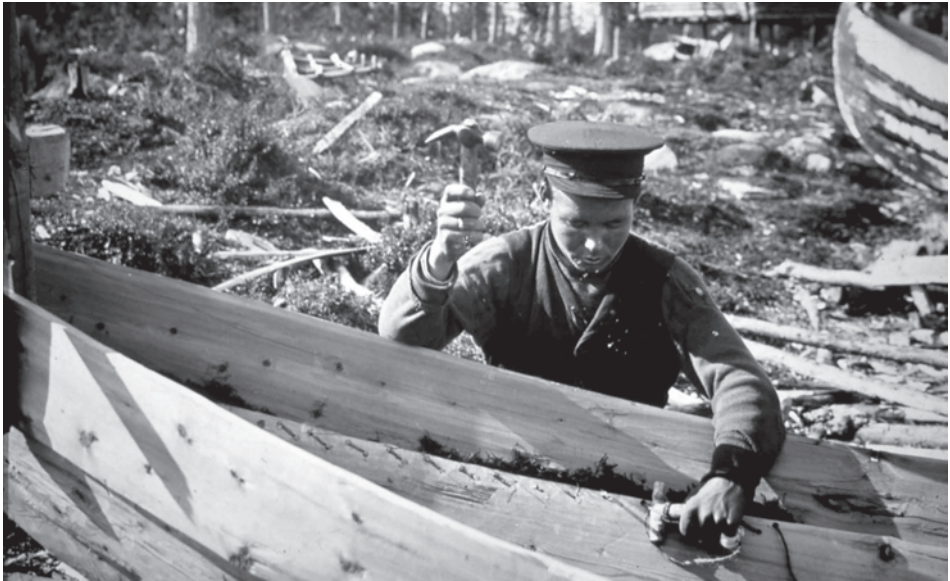
Fig. 5 A Skolt Sami boatbuilder in Nuotjaur (Notozersk) on the Kola peninsula wields a mallet-like tightening instrument lashing his boat planks together. (Photo: Gustaf Hallström, 1908 / Nordiska museet, Stockholm)
