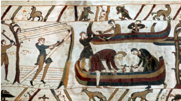
Fig. 61 Detail of the Bayeux tapestry dating from the 1070s, illustrating the two main processes of shipbuilding, the cutting of the trees in the forest and the building on the shore.
