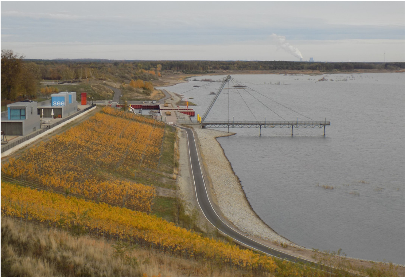
Fig. 4: The new lake in completion in the former open cast mine Meuro (Deshaies 2018)
