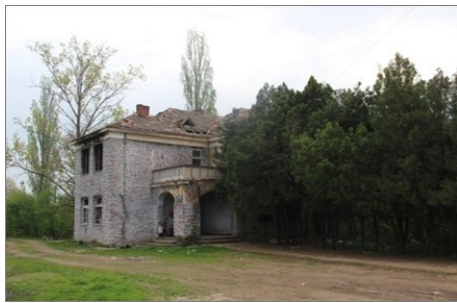
Fig. 4 – Former commandment of the 21 st Tanks Regiment
