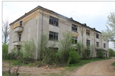
Fig. 5 – Abandoned barrack of the 21 st Tanks Regiment
