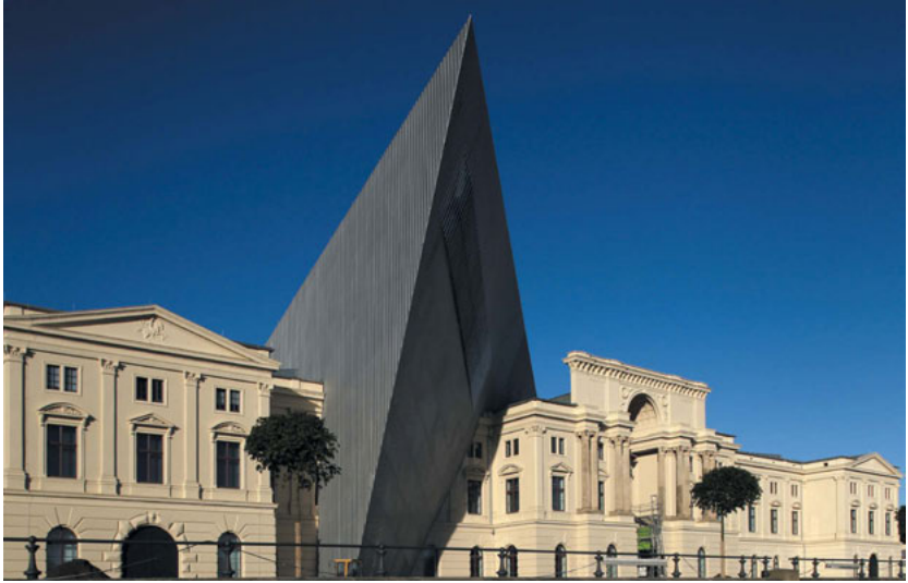
Military History Museum of the Bundeswehr, Dresden, exterior facade © MHM, Ingrid Meier
