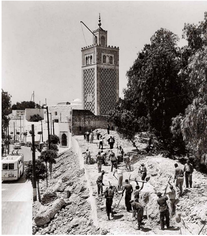
Figure 9 Demolition of the Walls and Barracks of the Kasbah
