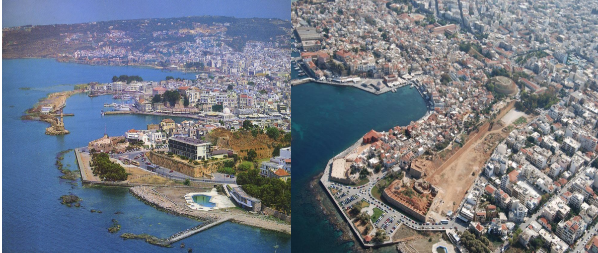
Figure 4-The hotel in the west bastion that was demolished in 2007.
