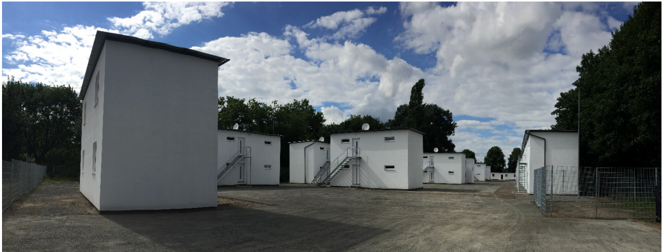
Figure 8. A purpose-built refugee accommodation compound for 200 people. The wooden-made structures resemble the design of modular container-villages and consist of two-floor structures with 2–4-person apartments. Source: author.
