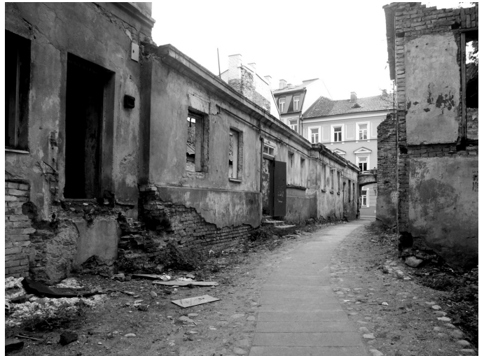
Photo 3: Dozens of buildings are only uninhabitable ruins. Photo: STANDL 2003
