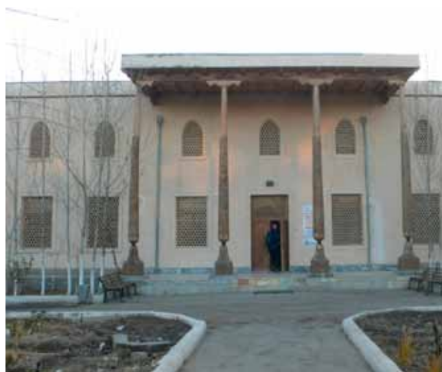
Project office at the compound of Urgench State University, Uzbekistan
