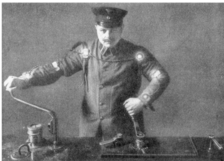
Tram driver with affixed white dots which facilitate the photographic registration of his movements. (Source: Tramm 1921.)
