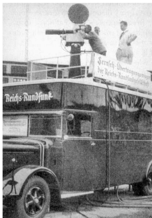
Electronic storage television pickup camera from Telefunken on the roof of the German pavilion at the Paris Exhibition of 1937 (In: Fernsehen und Tonfilm , No. 6, 1938).
