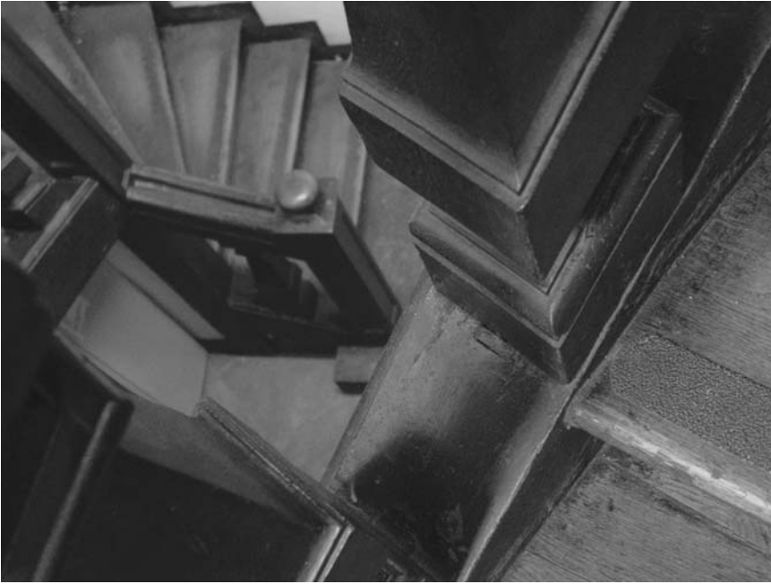
FIGURE 10 Spiralling staircase; photography © N. Gelijsteen.
